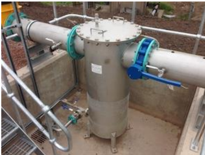
Figure 13: Condensation trap in a large biogas plant
