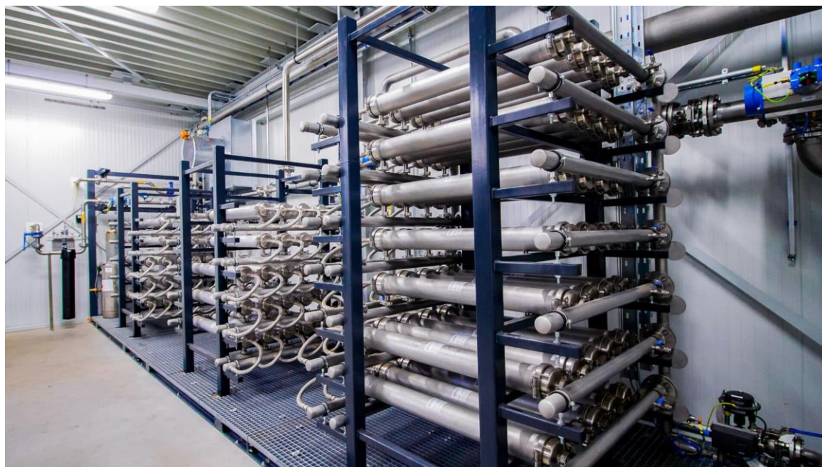
Figure 16: Example of biogas separating membrane filters
