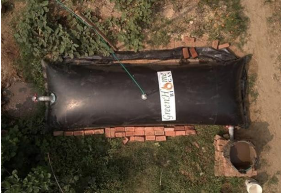
Figure 4: Membrane digester
